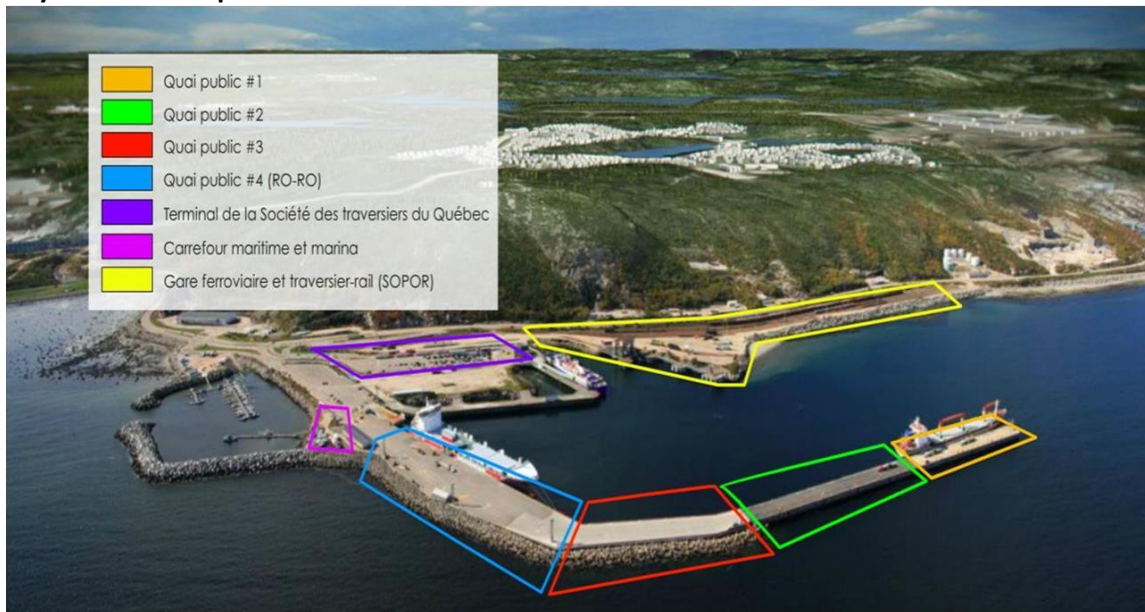
Figure 4. Technical description of berths at the Multi-User Terminal
